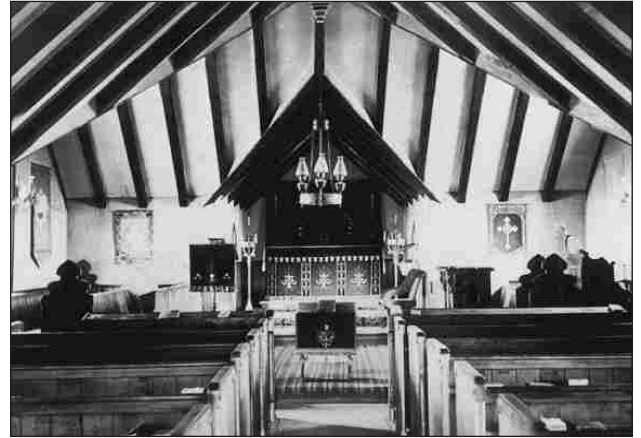
Interior of Church
